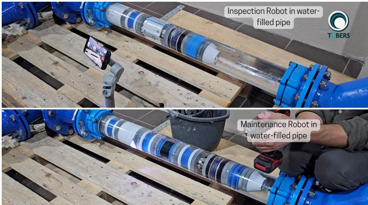
Figure 21: Inspection Robot and Maintenance robot operating under wet conditions, fully immersed in water.
